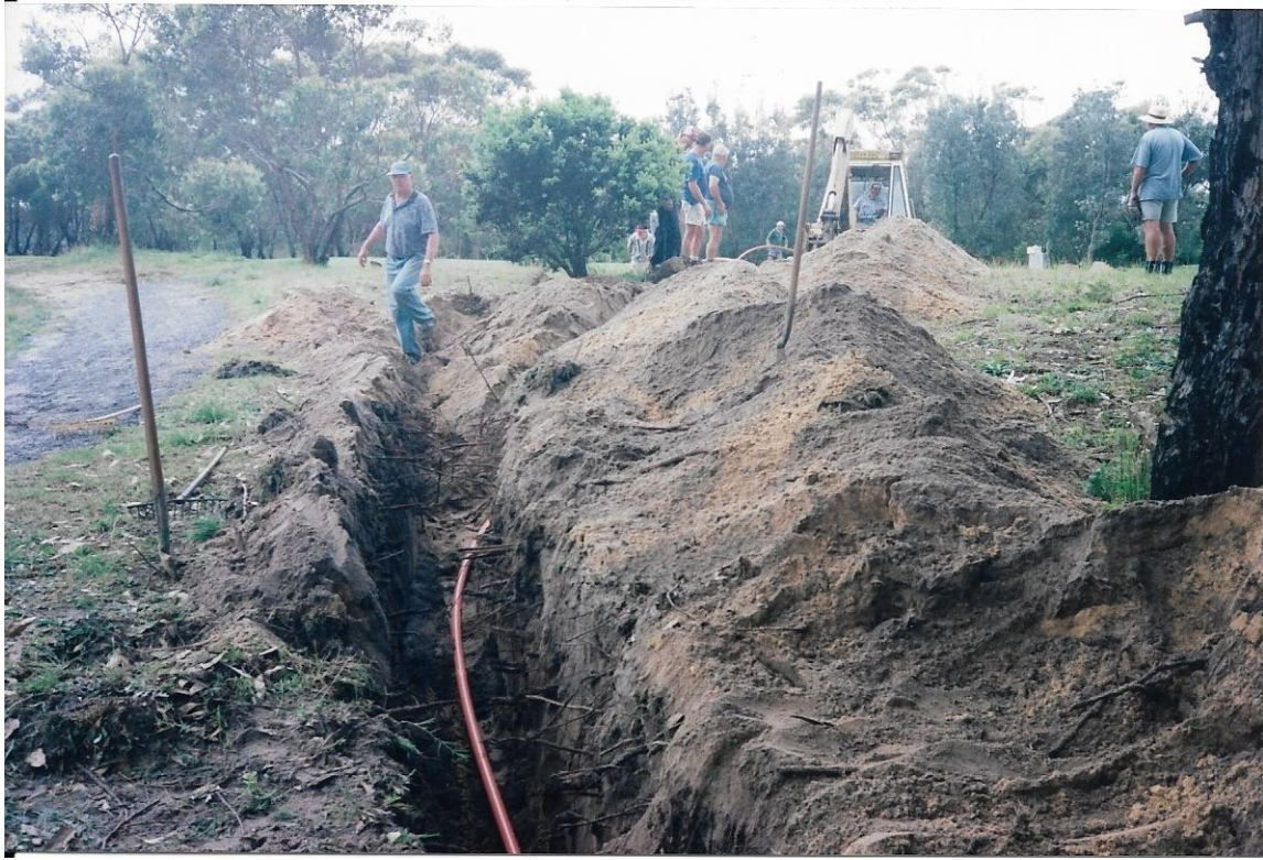
Laying power cable to pump shed 13 th green.
