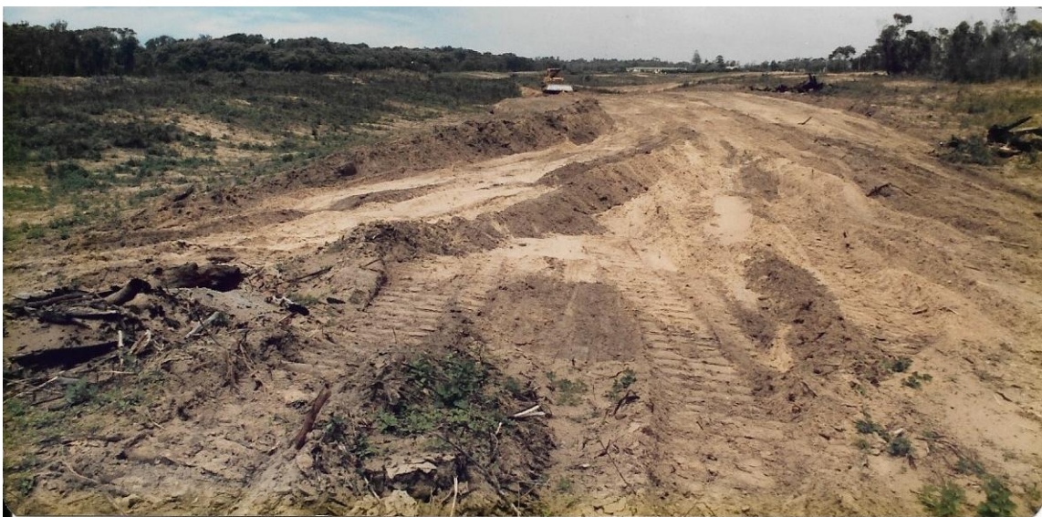
10 th fairway looking south – note size of storm water pipe
