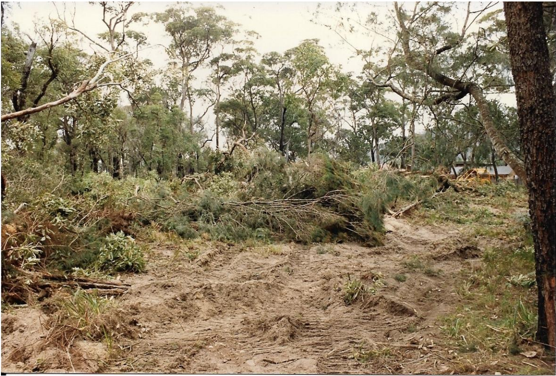
Early survey and clearing near Lovegrove Street
