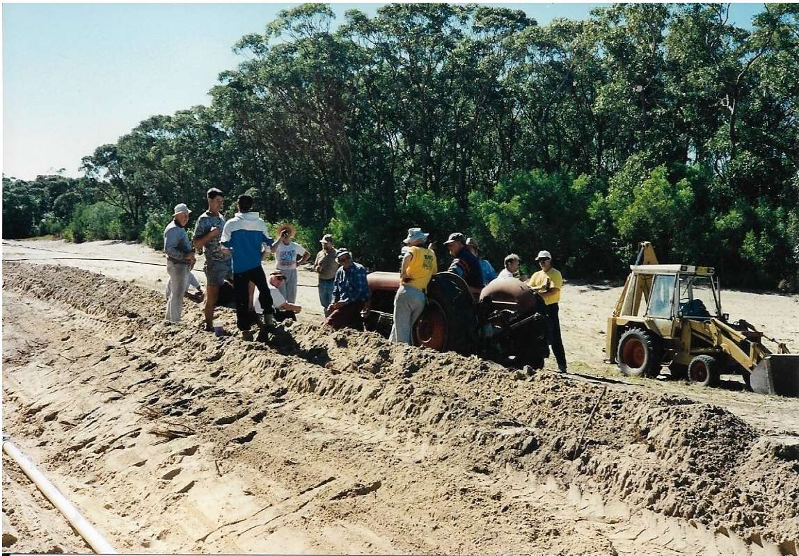
Irrigation pipe installing on 16th
