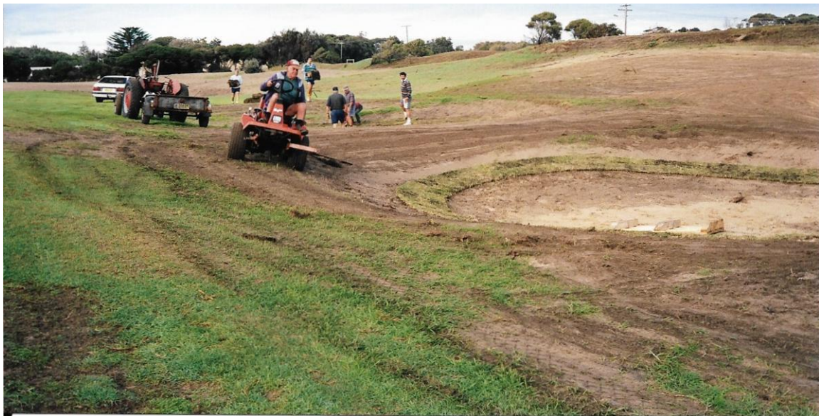
The bunkers on the 10 th – now filled in.
