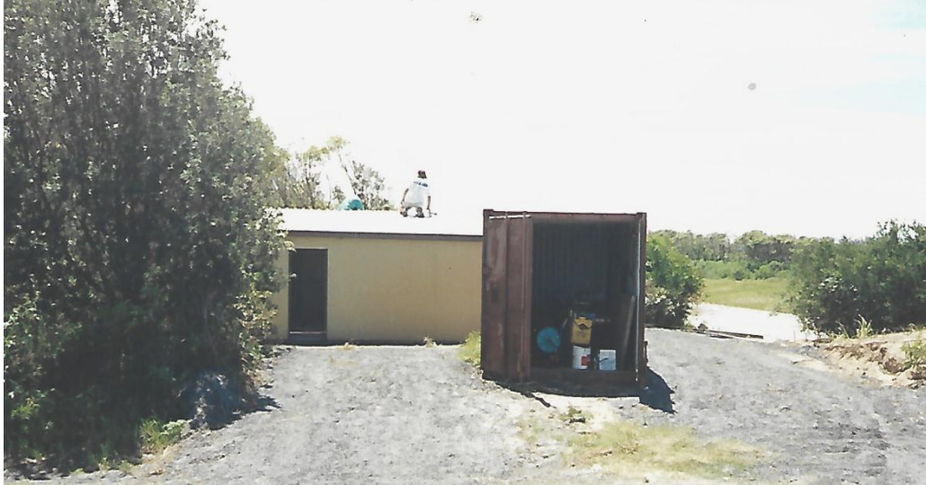
The second clubhouse being constructed
