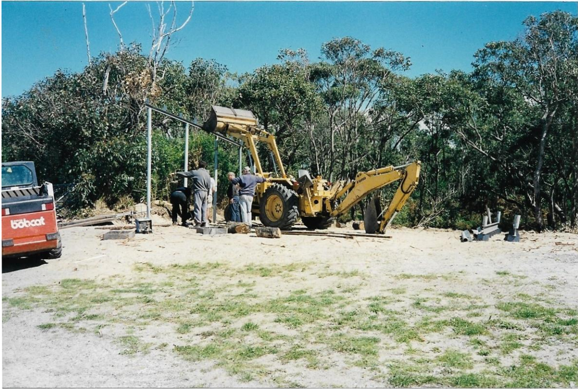
Starting the machinery shed
