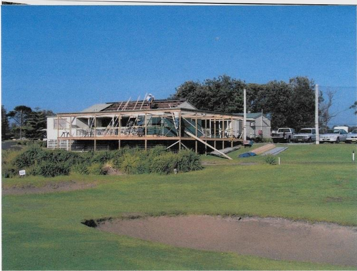
Adding veranda and re-roofing
