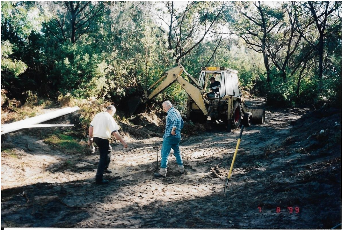
Terry Lillie, Cec. Montgomery & Alan Beveridge sinking spear points - Cec's first job after joining the Club.
