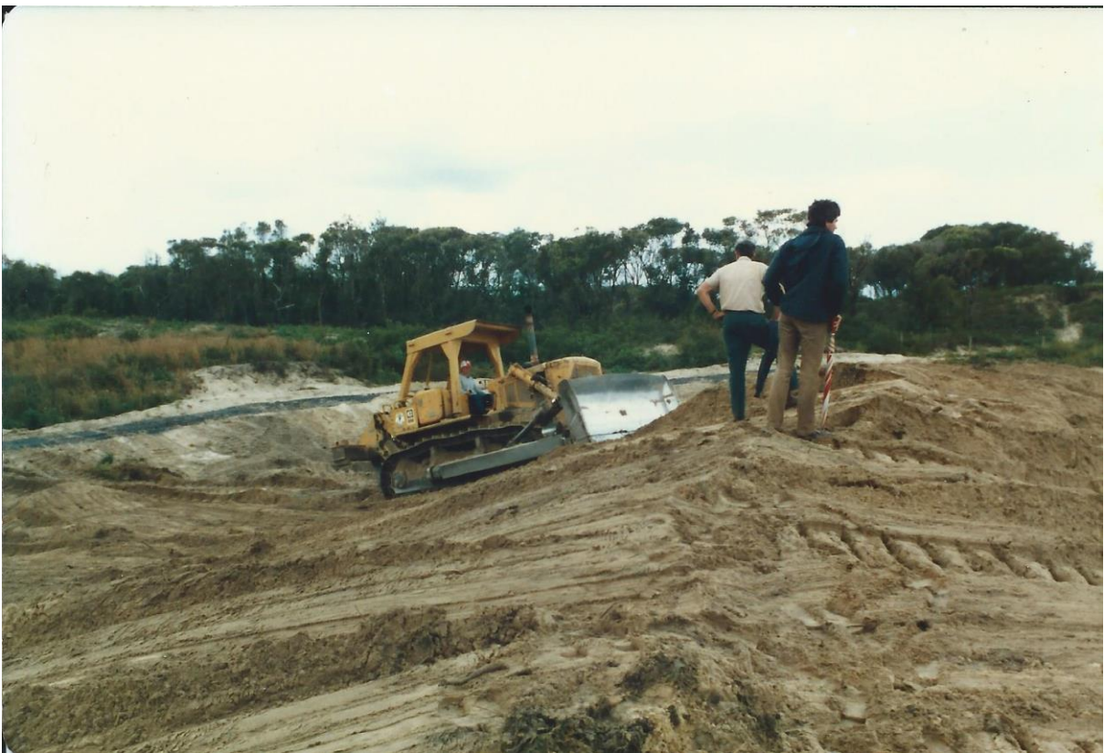
Creating the 12th green - Ken McKay with Council dozer
