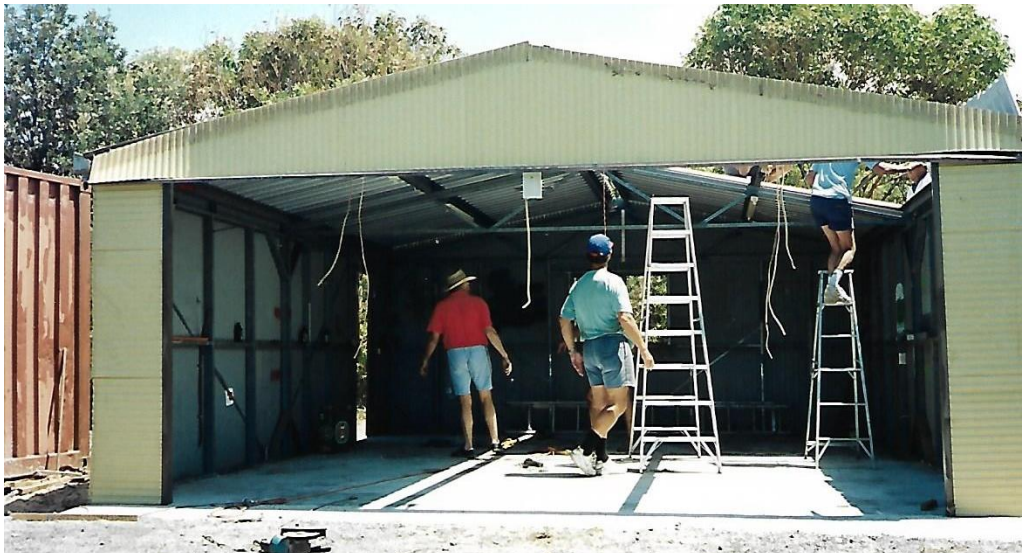
1996 - The third clubhouse being built next to Merv Jone's caravan (Below)
